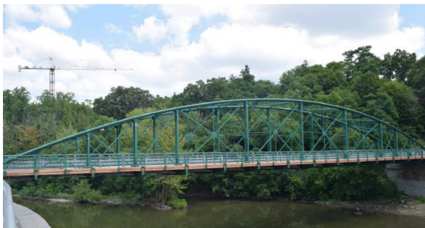
Figure 2. The Blackfriars Bridge, a bowstring truss bridge in Ontario, Canada
